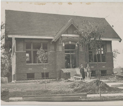
c. 1912 under construction
