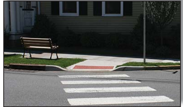
ADA Compliant Crosswalk Example
