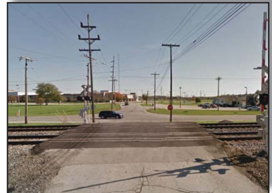
Railroad crossing on Madison Avenue
