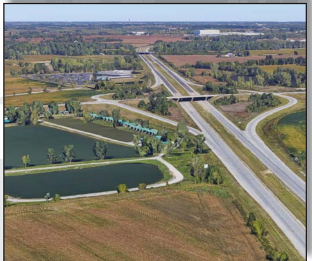
Interstate 69 at State Street
