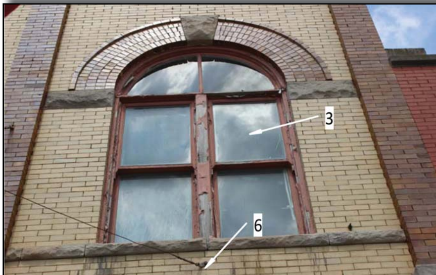
114 West State Street - Exterior Windows
