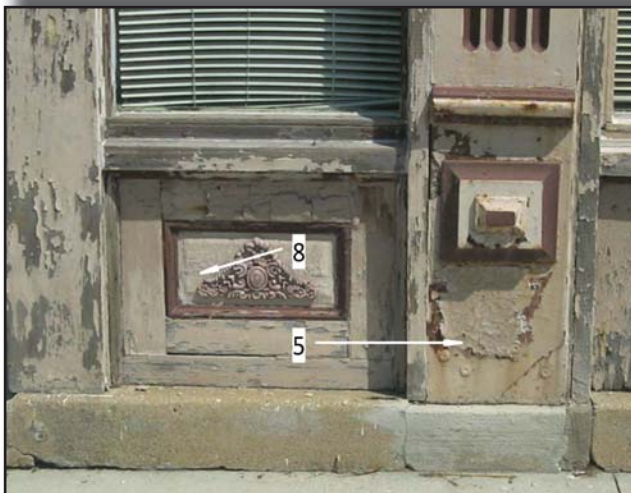
101 East State Street - Foundation
