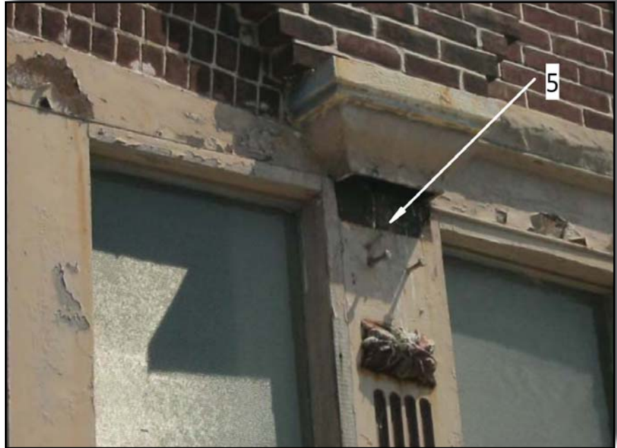
101 East State Street - Window Coping
