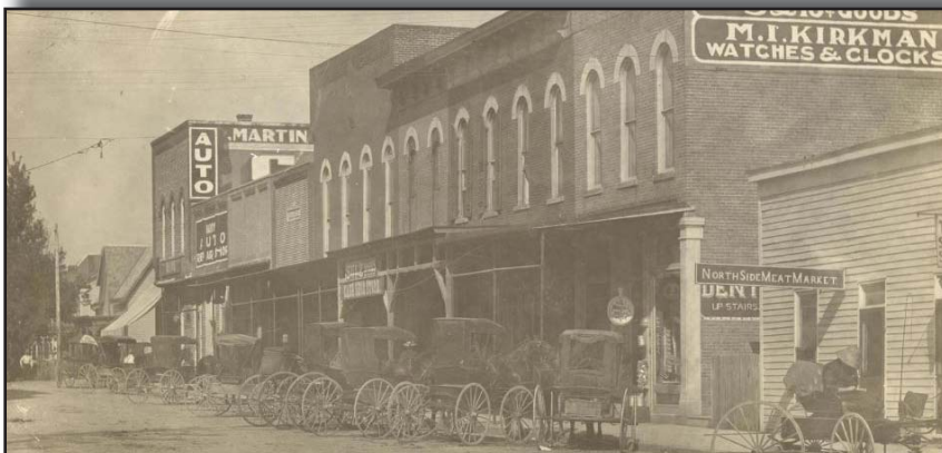
Historic Photo of State Street
