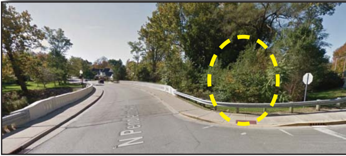
North - Pendleton Avenue (Guardrail to be removed)
