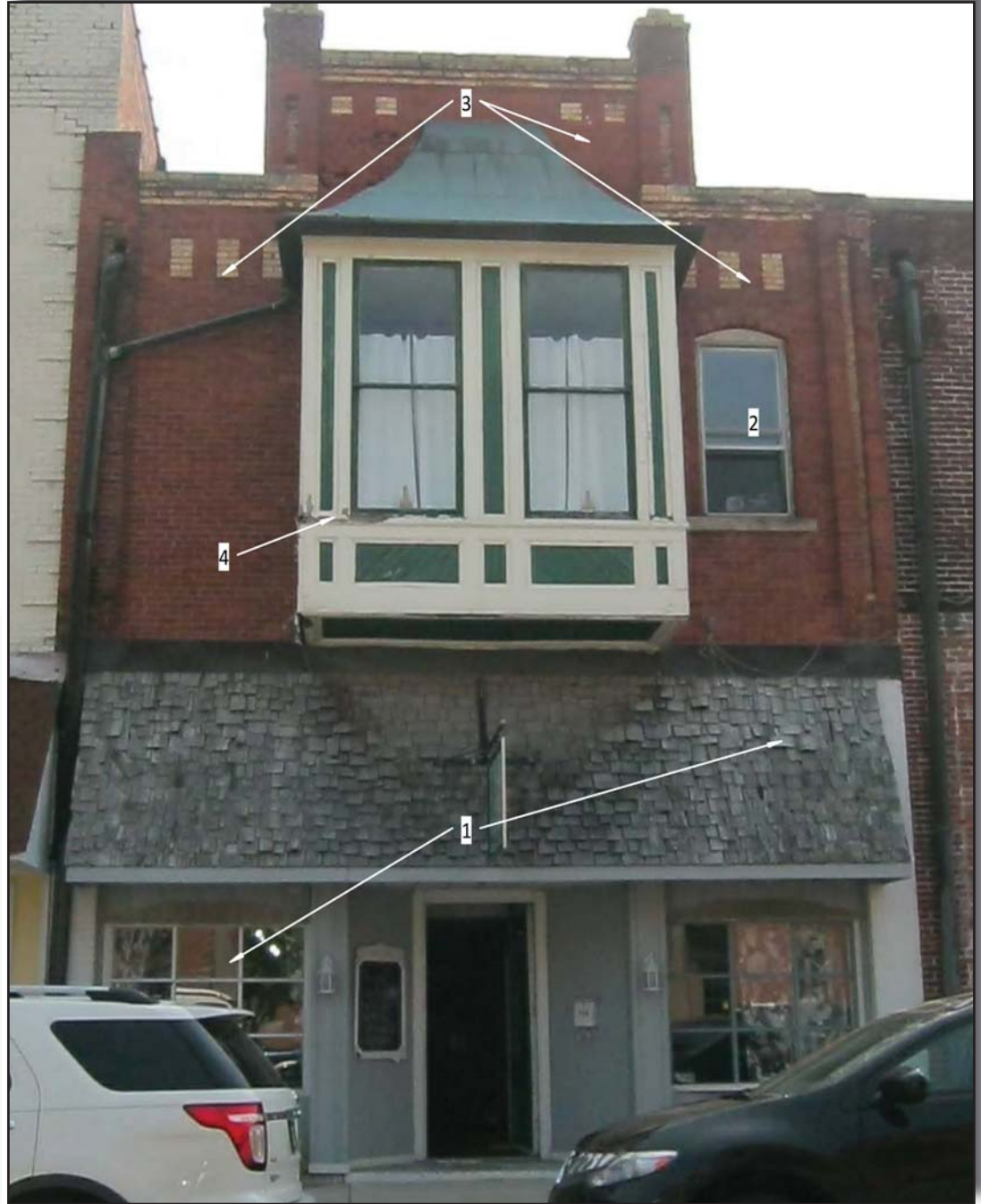
106 North Pendleton Avenue - Facade
