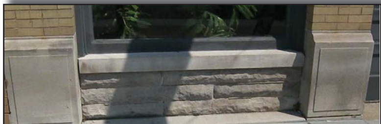
110 West State Street - Foundation
