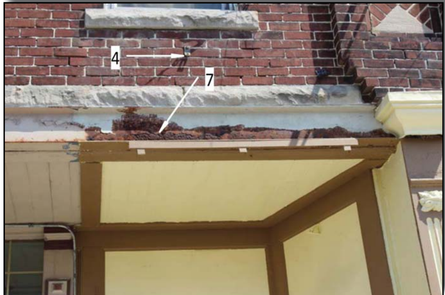
101 East State Street - Facade Entryway
