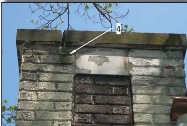
231 South Pendleton Avenue - Cornice
