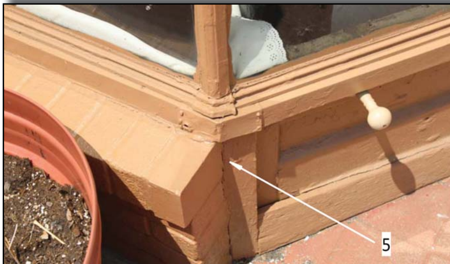
114 West State Street - Foundation
