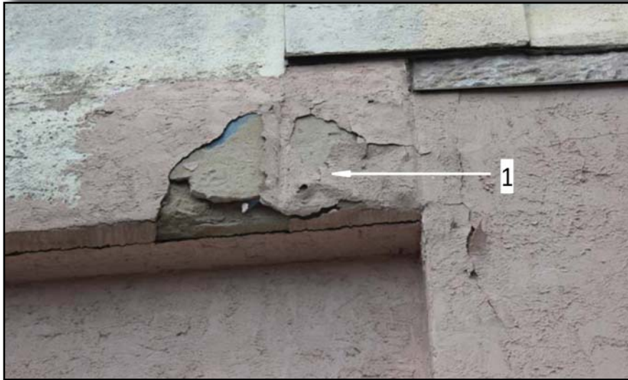
132 West State Street - Facade Masonry
