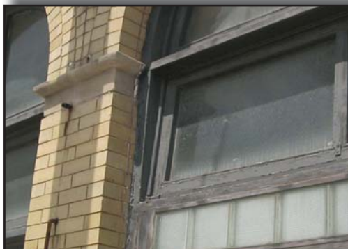
110 West State Street - Exterior Windows
