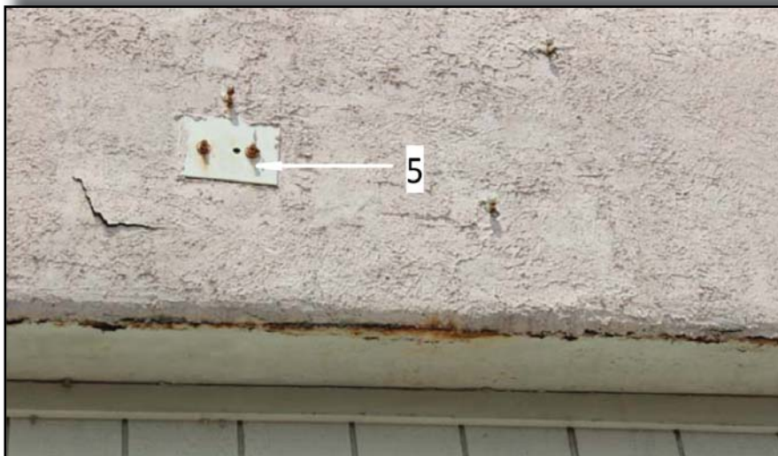
132 West State Street - Facade Masonry
