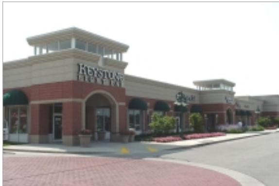
This structure uses multiple materials and a variety of details including changes in plane and windows. It also creates well-defined entries. The pedestrian scale of the arcade across the front is also a key feature.
